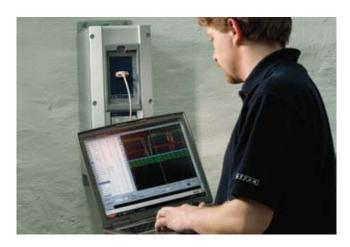
Emotron VFX offers easy programming and commissioning. Up to four parameter sets can be used and parameters are loaded to/from the variable speed drive by connecting an RS232 cable directly to the front.
